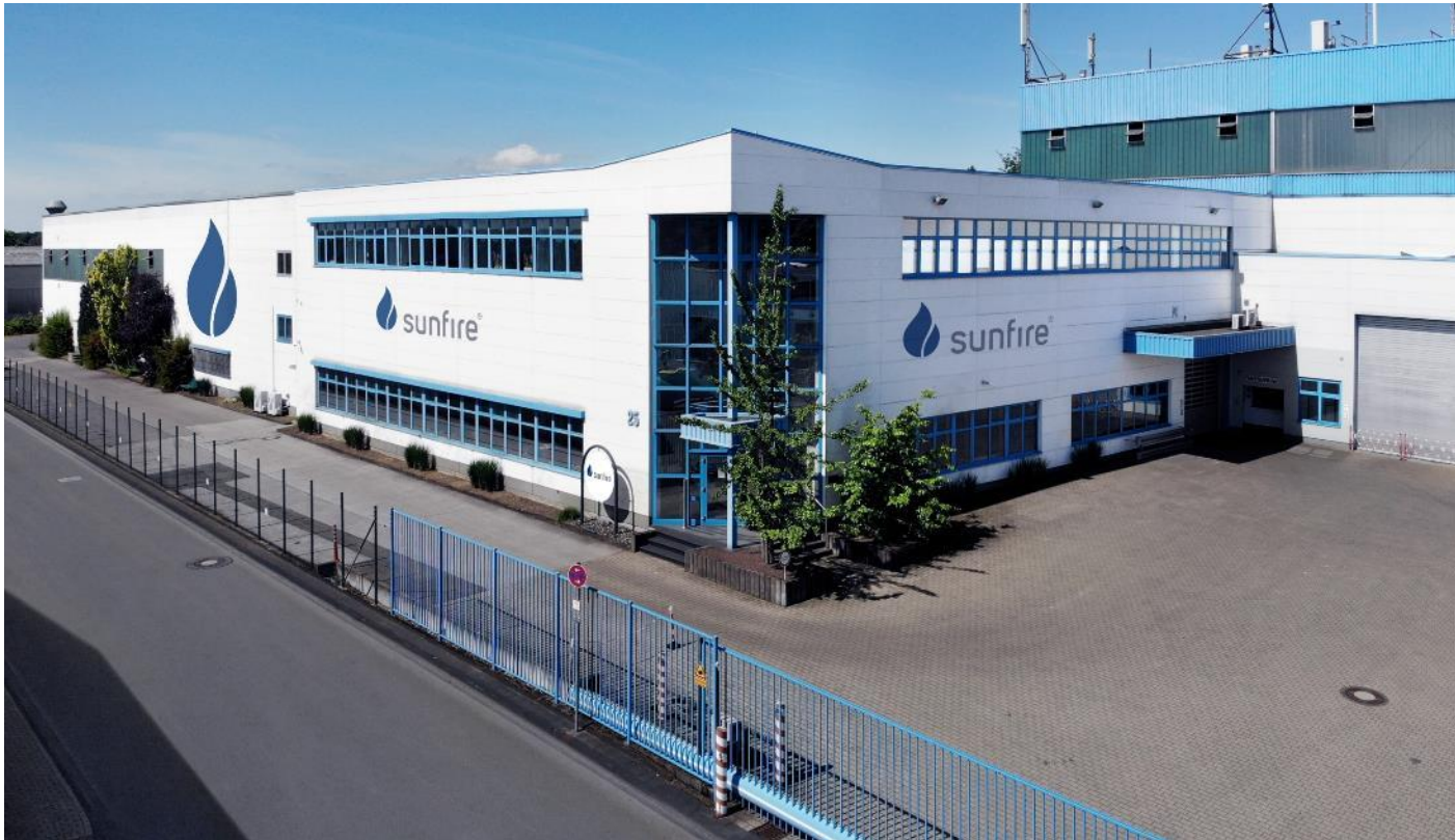
Sunfire's Galvancis facility for alkaline electrolyzer production in Solingen, Germany
